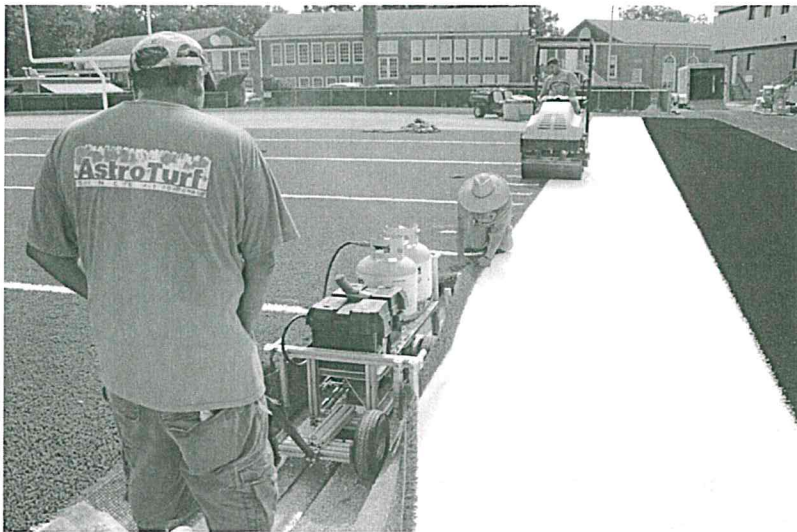
View of AstroFusion™ heat/pressure seaming system, which is exclusive to AstroTurf systems.
