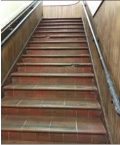
Stairway trip hazards.
