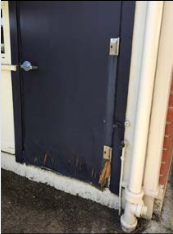
Water damaged door.
