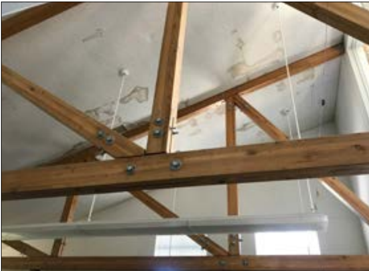
Ceiling damage from roof leaks.
