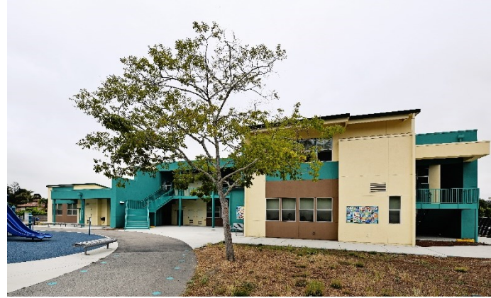
SOQUEL UNION ELEMENTARY SCHOOL DISTRICT SOQUEL ELEMENTARY SCHOOL NEW TWO-STORY CLASSROOM BUILDING
