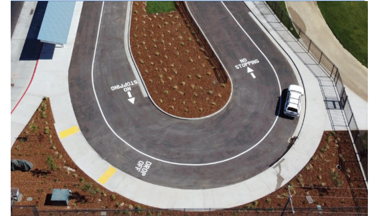
FAIRFIELD-SUISUN UNIFIED SCHOOL DISTRICT DOVER ELEMENTARY SCHOOL NEW DROP-OFF AREA & PARKING LOT
