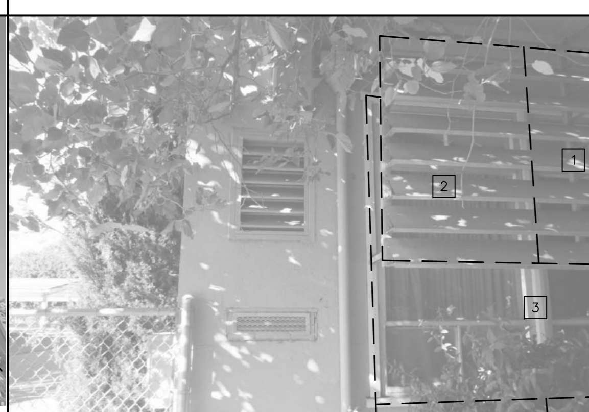
19 WALL, WINDOW & SHADE DEMO SOUTH WALL
