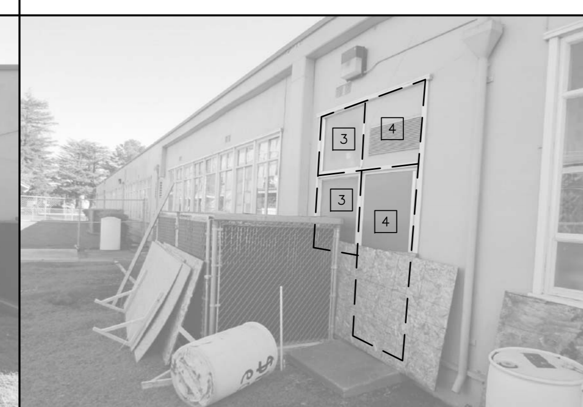
16 PREP ROOM DOOR/WINDOWS NORTH WALL
