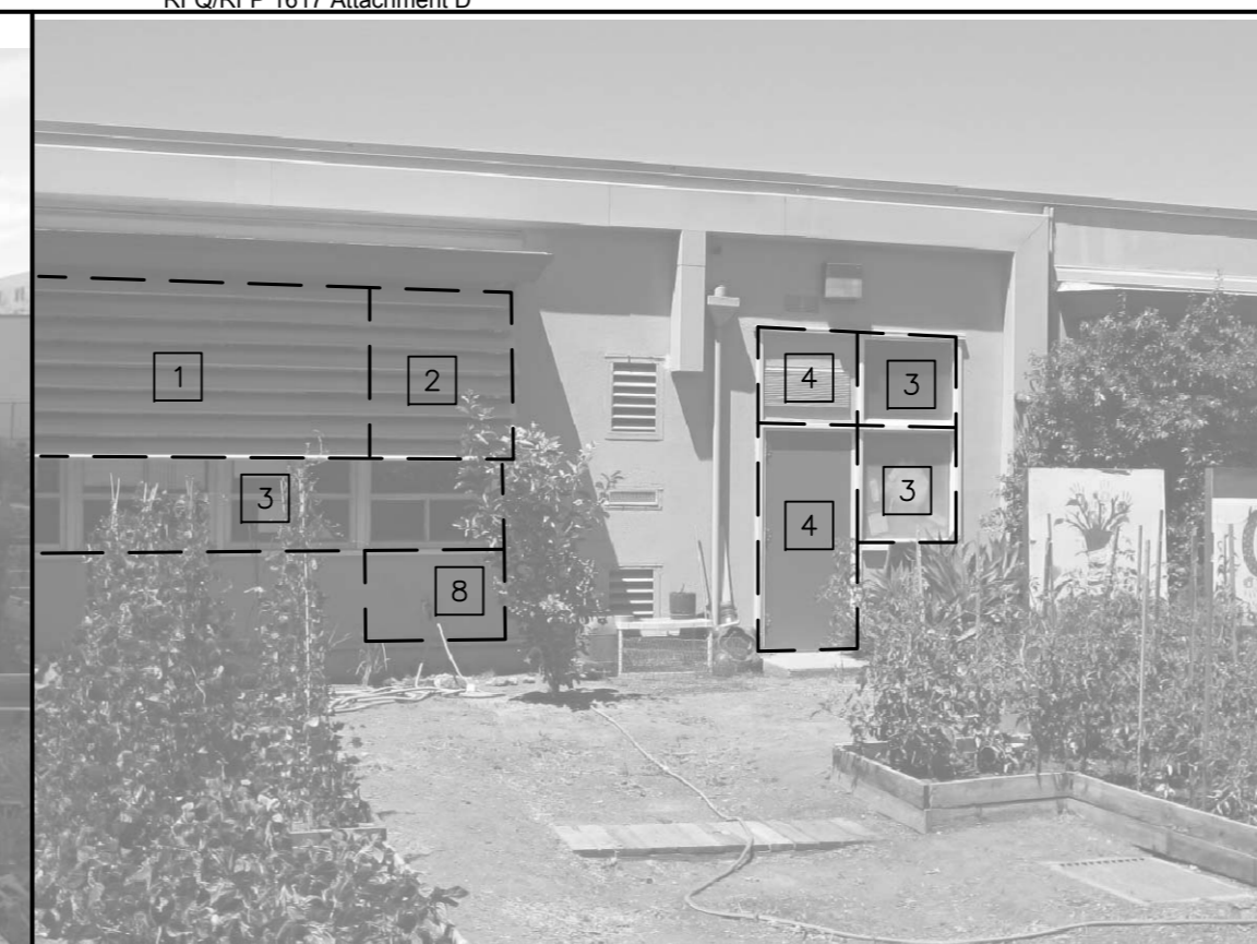
22 DOOR/WINDOW & SHADE DEMO SOUTH WALL
