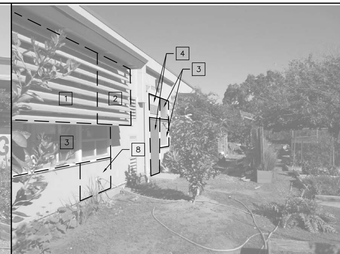
21 DOOR/WINDOW & SHADE DEMO SOUTH WALL
