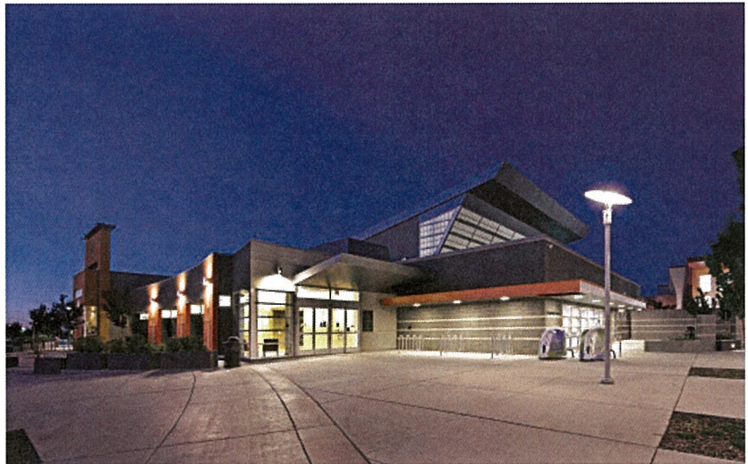
North Natomas Joint-Use Public Library Sacramento, CA
