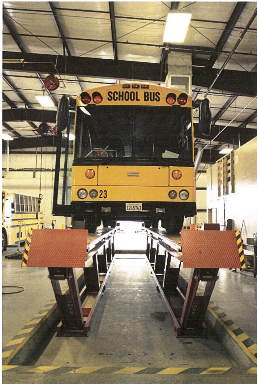
Yuba City USD Bus Maintenance Facility Yuba City, CA
