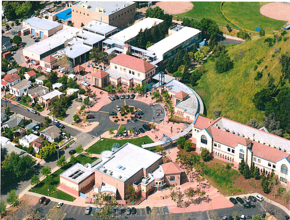
Alhambra High School, Martinez Unified School District
