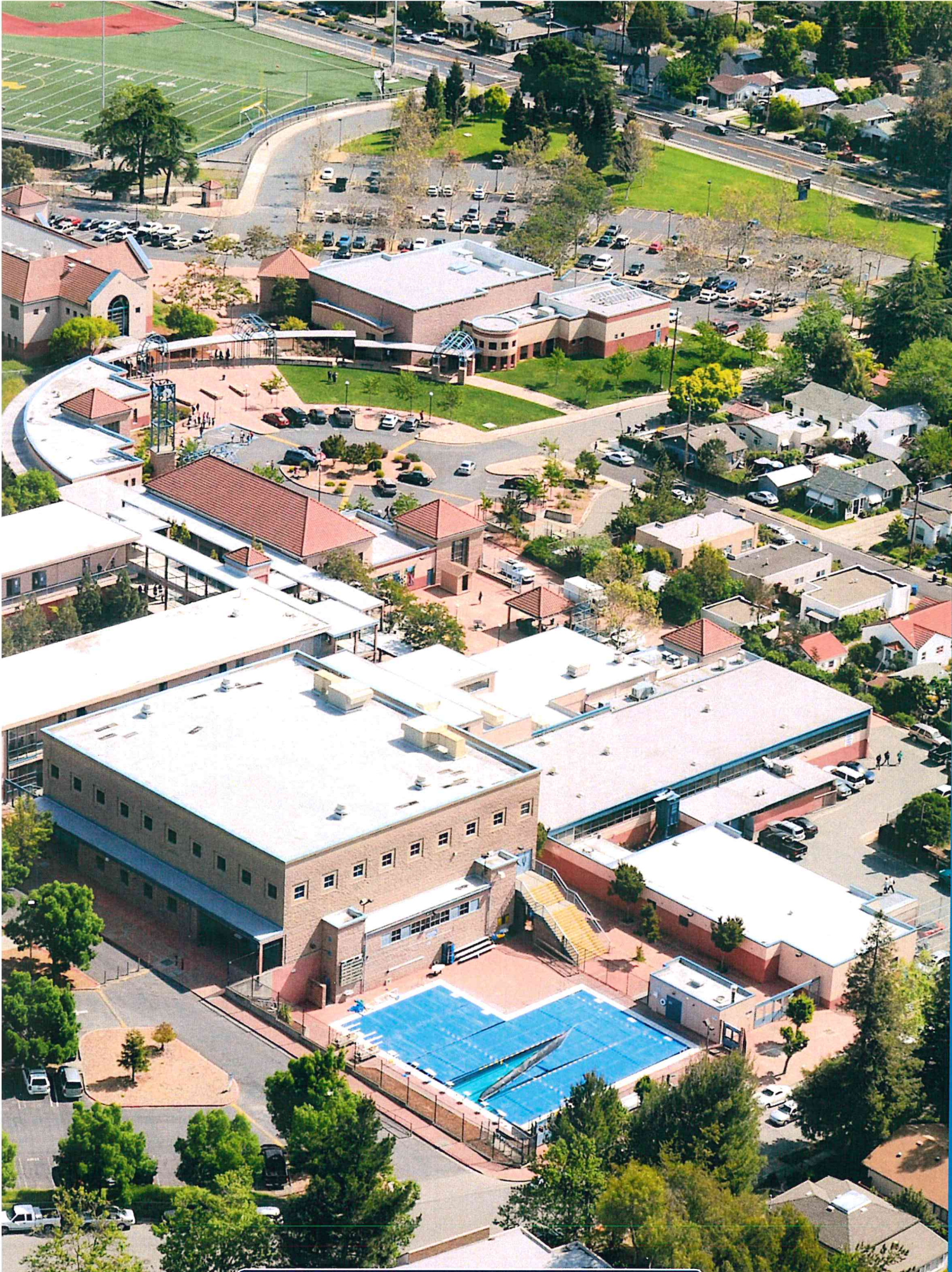
Alhambra High School • Martinez Unified School District
