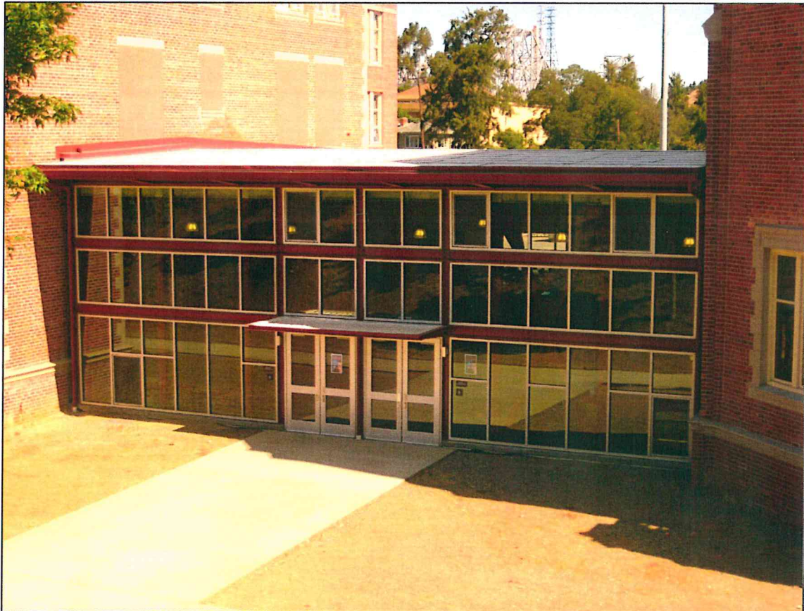
John Swett High School, Building D, John Swett Unified School District
