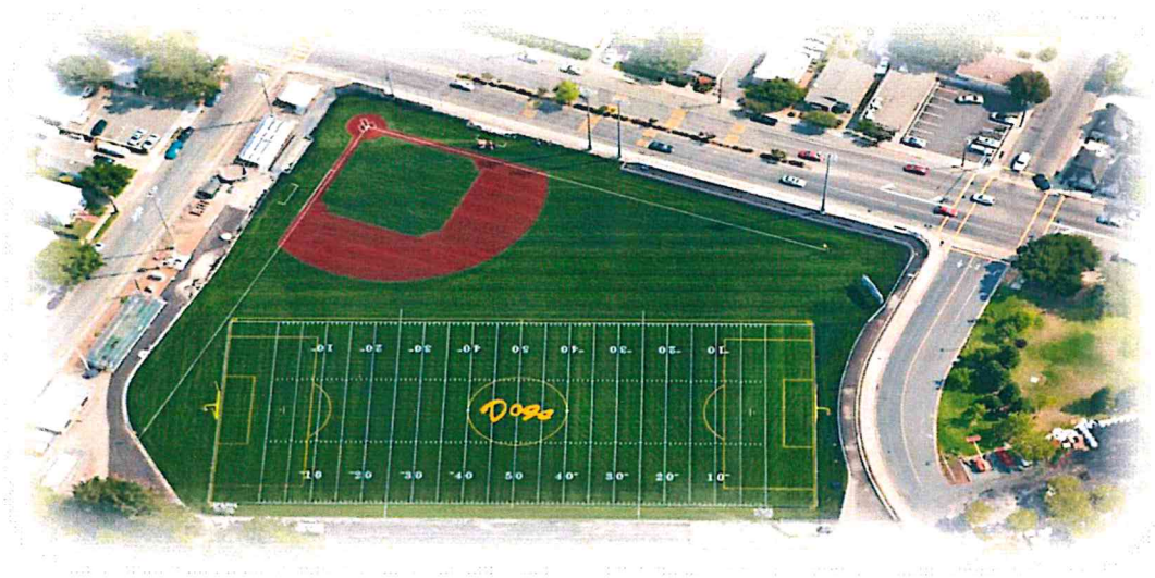
Alhambra High School, Martinez Unified School District
