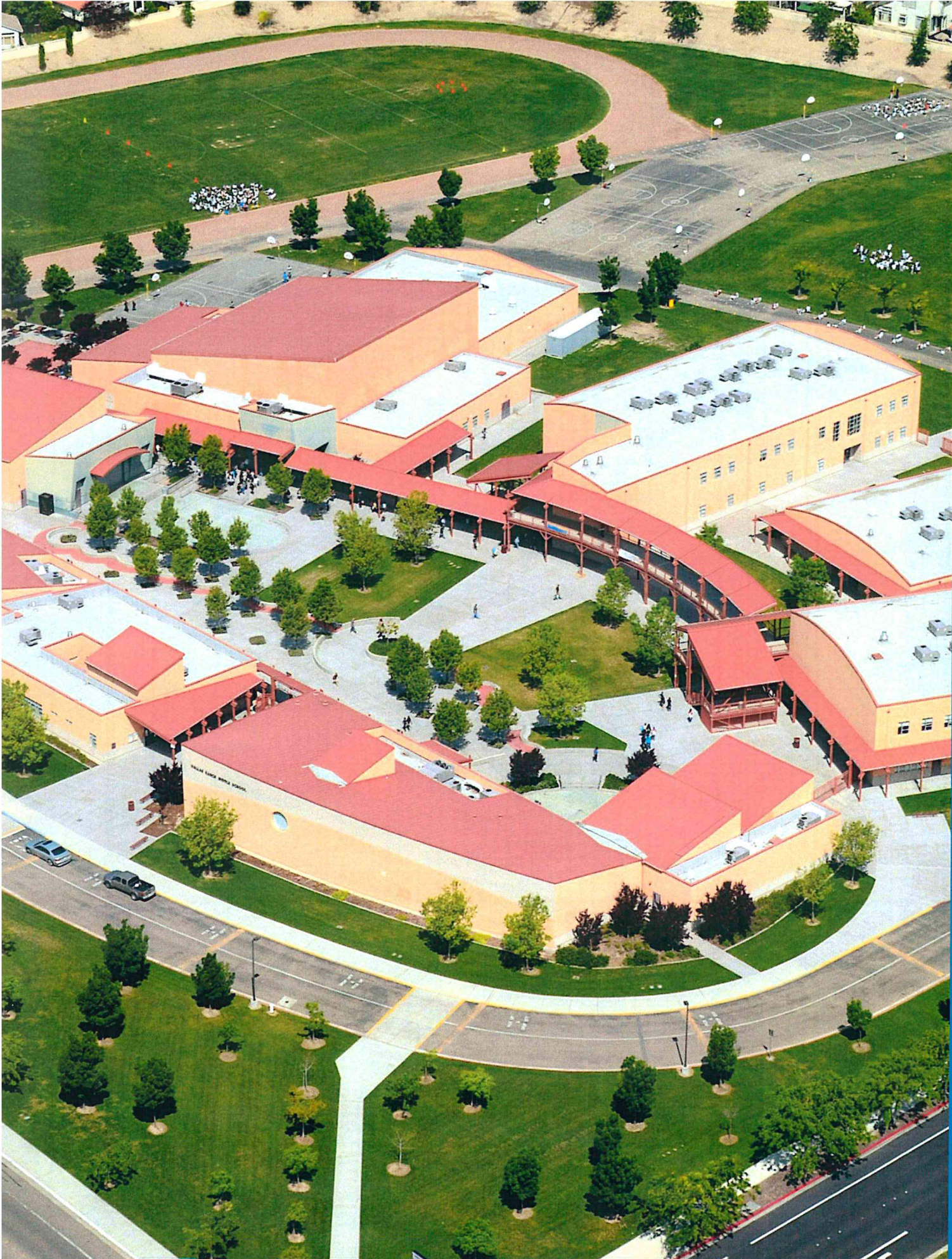
Dallas Ranch Elementary School • Antioch Unified School District
